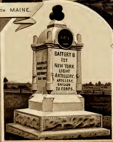
NEW YORK BATTERY B. HANCOCK AVENUE.
